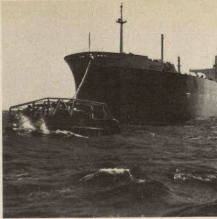
The present trend in offshore port construction is to couple tankers to single-buoy moorings miles offshore. Crude oil is unloaded at the mooring and pumped inland for treatment and storage. (Photo: J. Ray McDermott & Co., Inc.)
