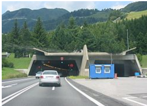
St. Gotthard Road Tunnel
